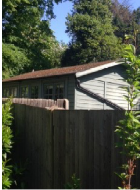
Photo 5 – view of boundary fence from within rear garden of no.4
