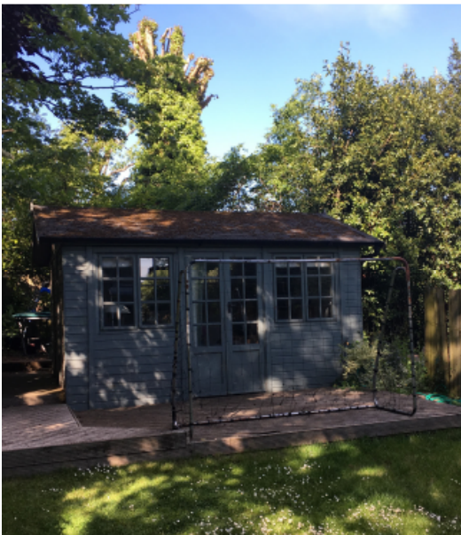
Photo 6 – existing outbuilding in rear (no.4a)
