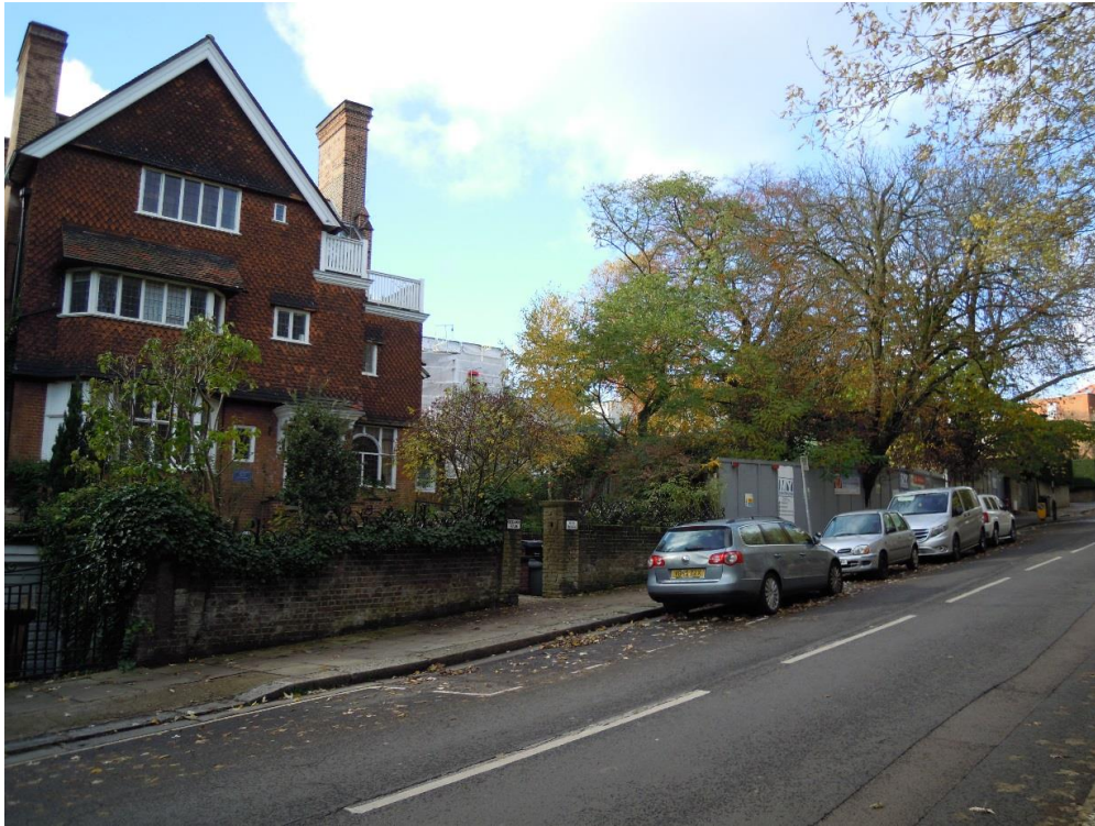
1. Looking north to southern end of site's frontage
