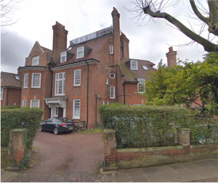
1. View towards front elevation of property
