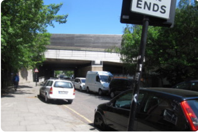
Figure 27: Camley Street bridge
