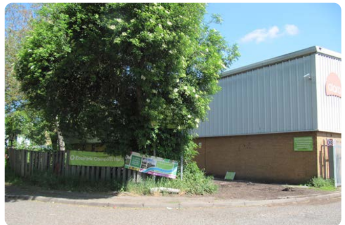
Figure 17: Compost Hub and Alara, 110-112 Camley Street
