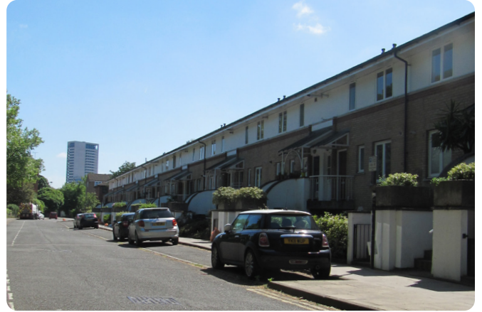
Figure 22: Row of terraces along Barker Drive
