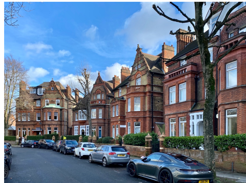
Lyndhurst Gardens. Properties are set back behind front gardens and are stylistically diverse. Common characteristics include bay windows, gables, and chimneys.
