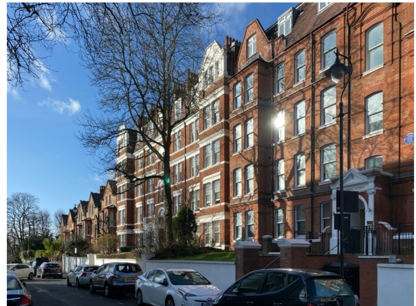
Common features of properties of all kinds include use of modulation (projection and recession of features), varied window styles including bays and dormers, open porches, gables, pitched roofs and chimneys.
