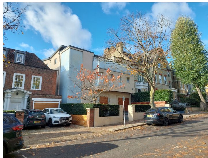
Distinctive examples of a Contemporary houses in the Conservation Area.
