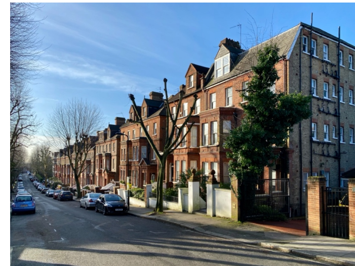
The Conservation Area is architecturally diverse, but with large groupings developed in a planned way. Enhancing the character or appearance is not about imitation, but high-quality site-specific design, complementing the
