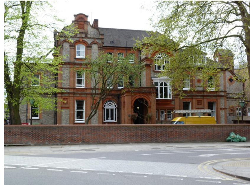
Grade II Listed No. 40 College Crescent is located at the southernmost end of the Conservation area. Use of grey and red Reading bricks with terracotta enrichment and continuous dentil cornices at floor level, with a Dutch gable.
