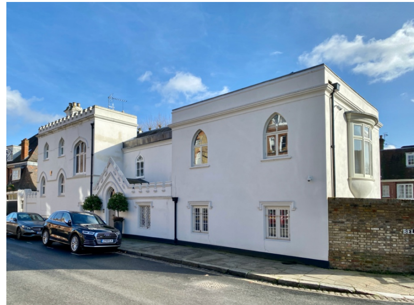
No. 5, Hunter's Lodge, in Belsize Lane, in a picturesque gothic style, contrasting with the wider character of the area.
