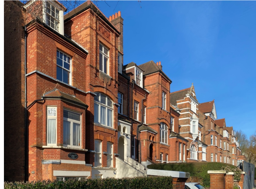
The townscape quality varies in different streets in the Conservation Area. Development should respond to the predominant townscape character in terms of height, scale, massing, gaps between buildings, and degree of setback from the road.
