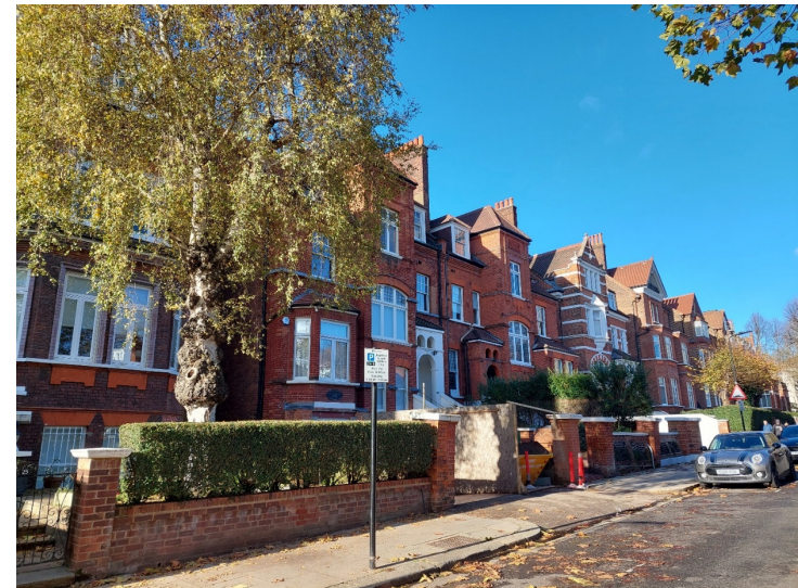
Newer development in Netherhall Gardens aligns with the scale and general townscape character of the road, without resorting to stylistic imitation.
