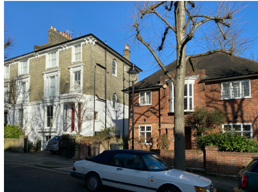
Eldon Grove. Different parts of the road were developed separately, creating group value to properties developed together in a similar style. This is typical of many roads in the Conservation Area.
