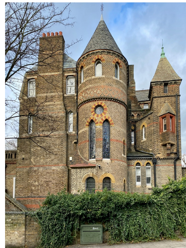
Gothic Revival property at the junction between Lyndhurst Terrace and Lyndhurst Road.
