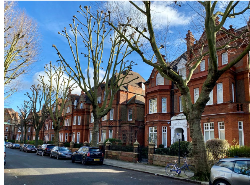
The area's verdant character includes buildings set back behind front gardens and street and garden trees.
