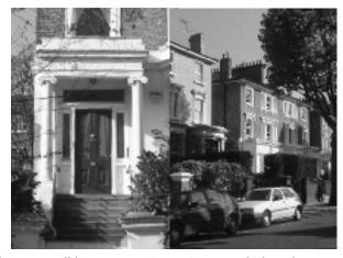
detailing around first floor windows. Chimney stacks on the party wall line are prominent. Some stacks have been reduced and many pots are missing. The villas are built in an attractive light buff coloured facing brick. Although many of the garden wall piers remain, original railings are missing and some front gardens have been opened out for car parking. A similar pair is found on the north side at Nos. 33 & 34 set amongst the listed 'artistic' housing.
