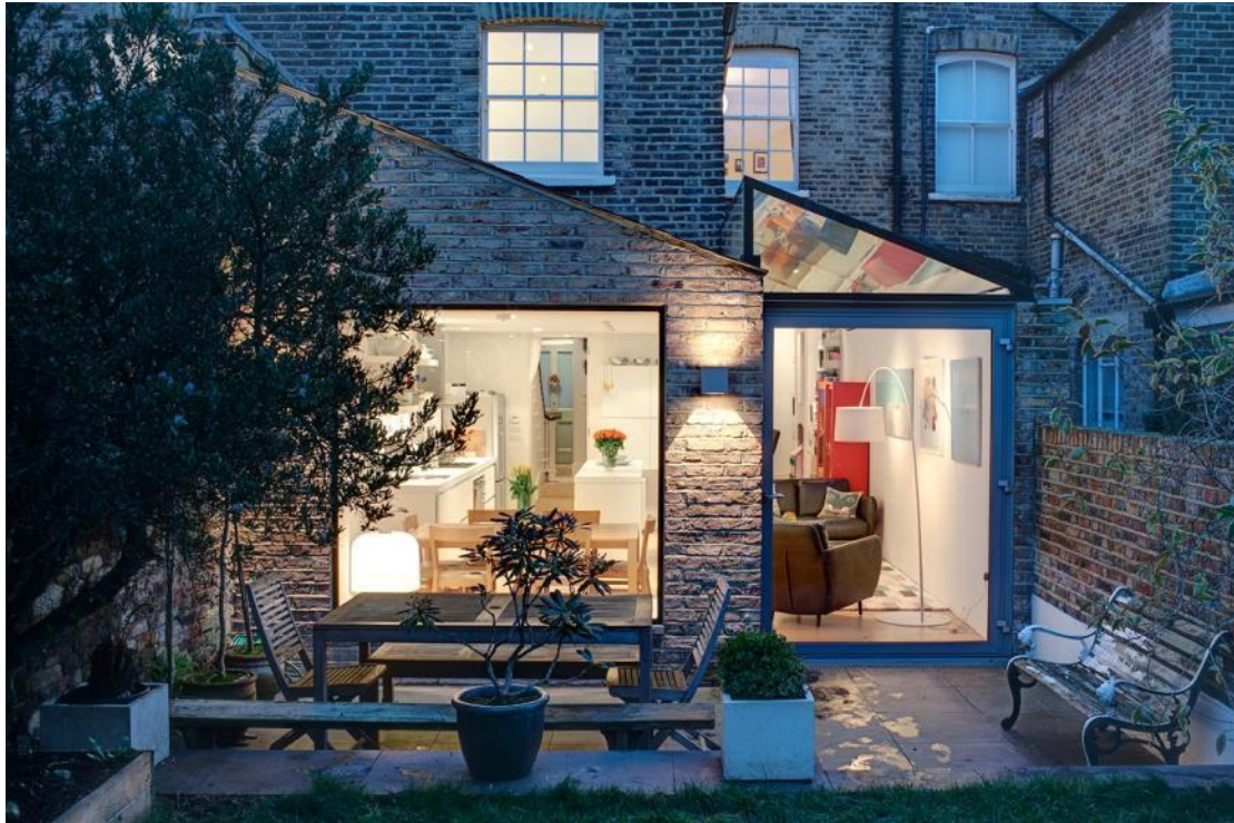
Ground floor extension, Chetwynd Road (architects: Cousins and Cousins; photo credit: Luke White)
