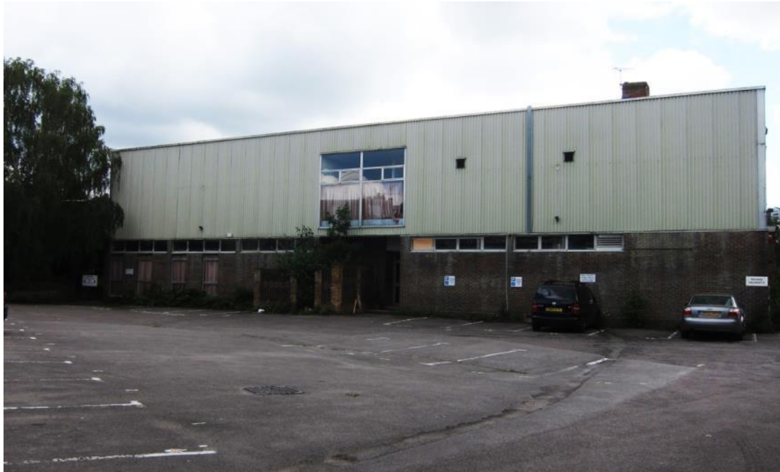
Mansfield Bowling Club (before demolition)
