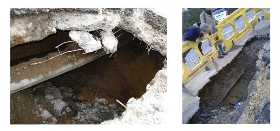
On the left is a photo of a large cavity uncovered under Heath Street, outside the Baptist Church. To the right is a sink hole that appeared in New End. These illustrate the erosion of a significant volume of silt from the Claygate Beds by the action of groundwater, causing subsidence, cavities and sink holes. This action is magnified when basement developments constrain and thus speedup the groundwater flow.
