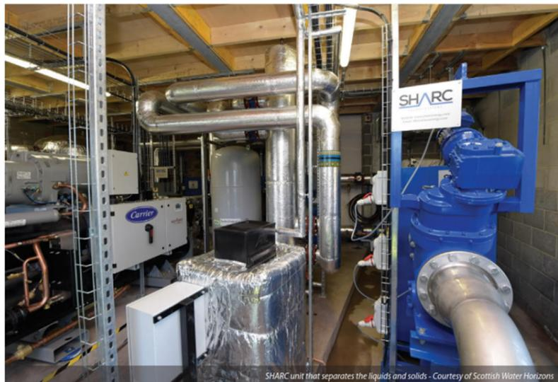
Figure 16 – Borden College Sharc Heat Exchanger and Filtration System
