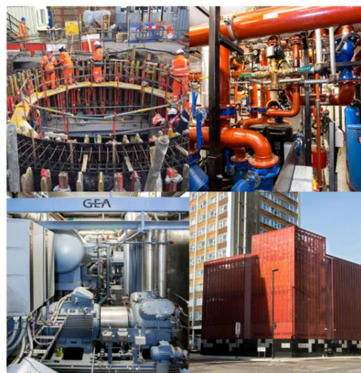
Figure 6 – Bunhill 2 energy centre GEA ammonia heat pump
