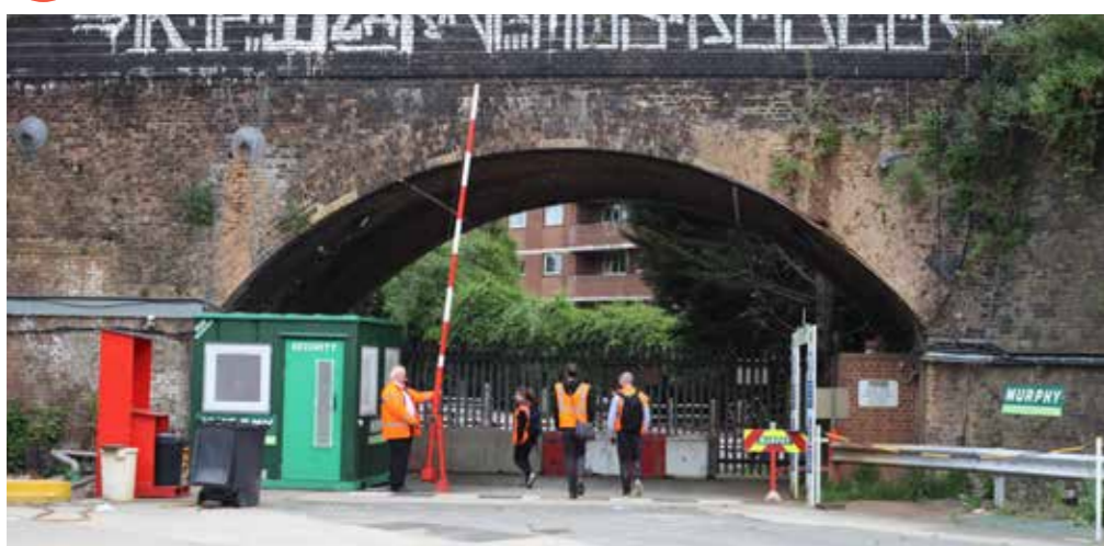
Constrained access into area
