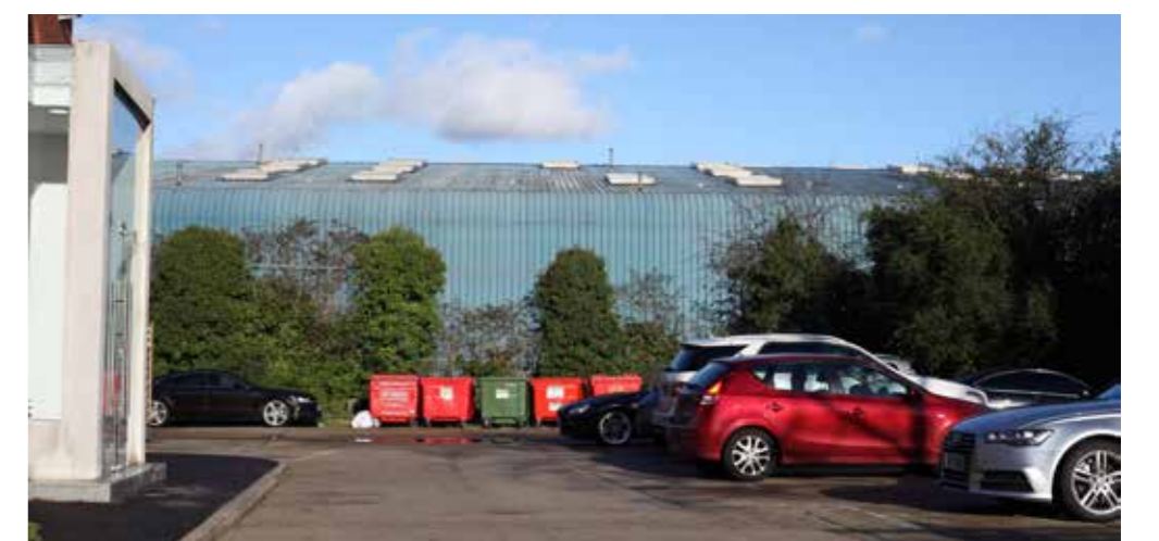
Poor quality buildings and public realm
