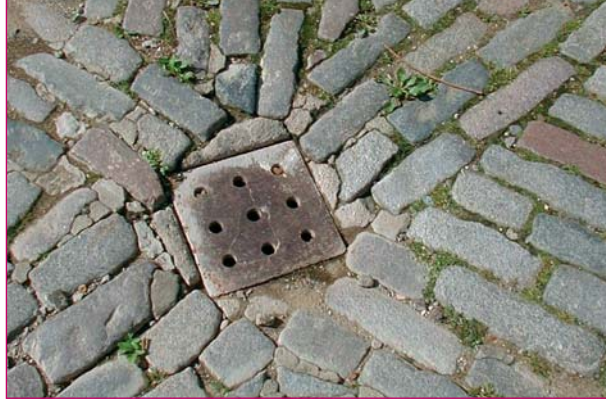
Setts used in traditional drainage techniques
