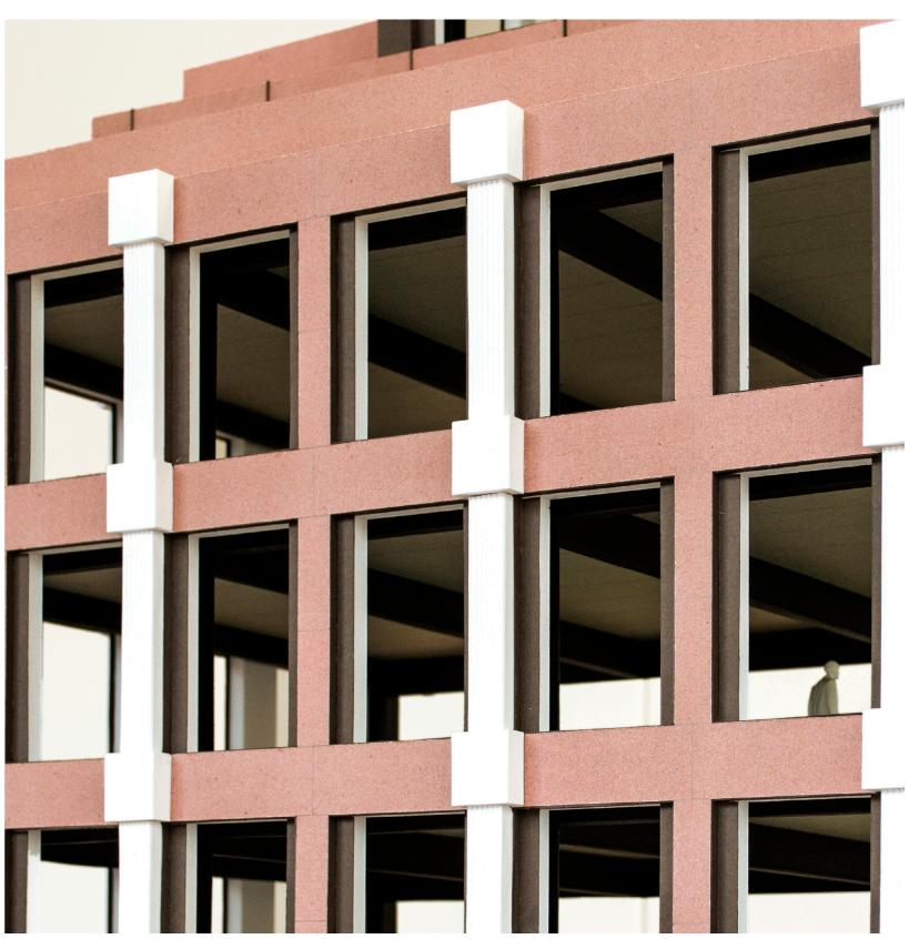
Model of the facade with sandstone spandrel panels, black metal window frames and pale precast concrete pilasters and capitals
