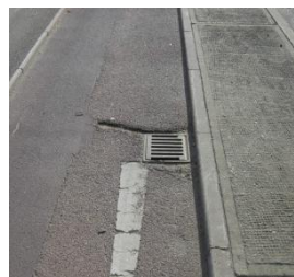
Figure 2.20 Maintenance issues for cyclists: surface quality
