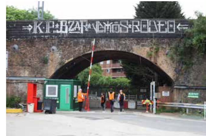
Constrained access points to both Murphy's Yard and Regis Road
