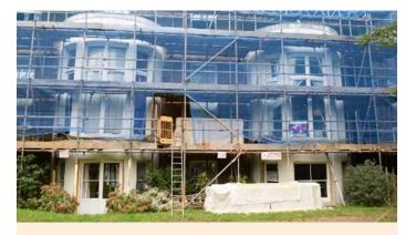
Camden launched a major retrofit project at **5-7 Belsize Grove estate**. The works include improved glazing, ventilation insulation, solar energy and low carbon heating upgrades and will improve the energy efficiency of **58 council homes**.
