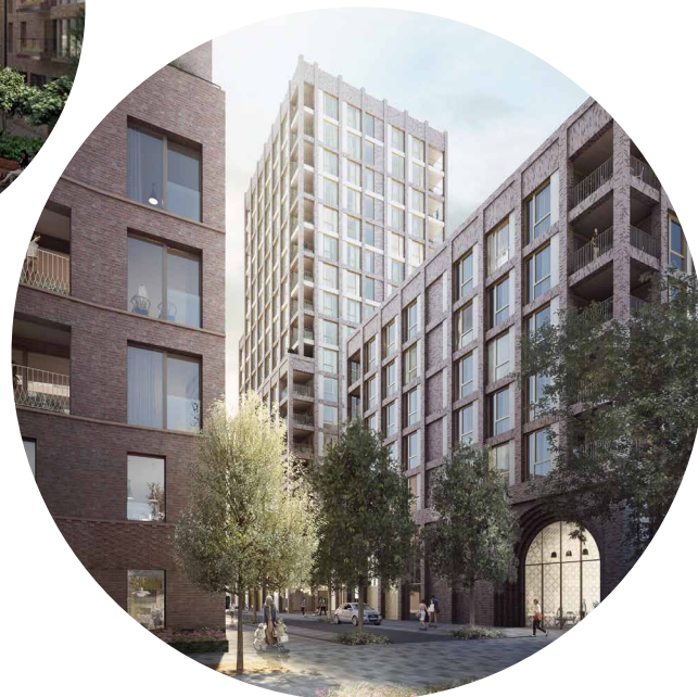
Agar Grove Plot B, Hawkins\Brown with Mae, LBC (Image: ForbesMassie) The development follows the principles of Passivhaus architecture, allowing for greater energy performance and cutting down fuel poverty.
