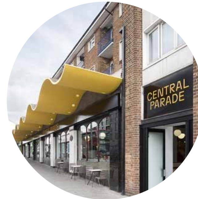
Central Parade, Walthamstow (Gort Scott) - Mixed-use scheme provides a bakery, café and events space, retail spaces and coworking areas with meeting rooms and studio units for up to 50 independent creative businesses. The basement includes rehearsal spaces and recording studios
